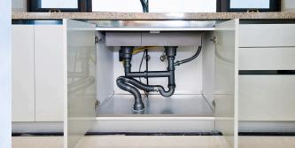
**Open cabinet doors to allow heat to get to uninsulated pipes under sinks and appliances near exterior walls.**
