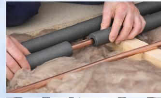
**Insulate pipes in unheated areas such as garages, attics, and crawl spaces.**
