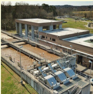
Treatment Plants 2 Wastewater Treatment Plants 2 Decentralized Treatment Plants
